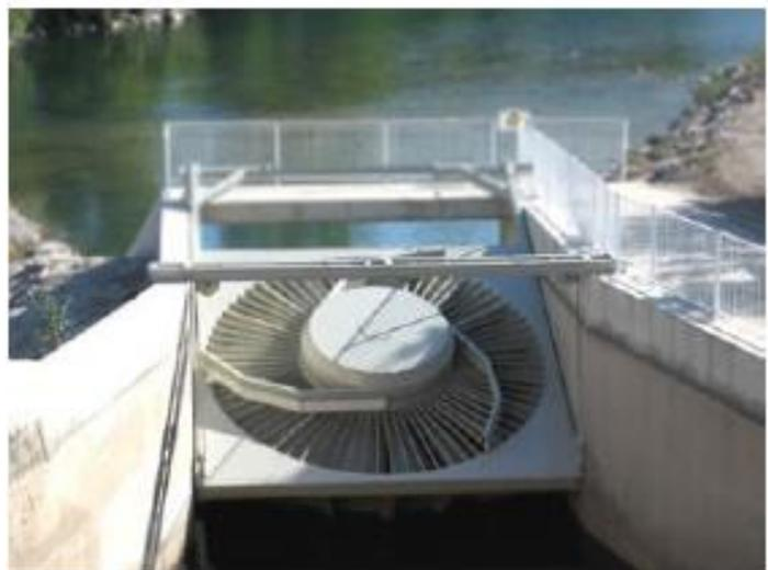
Figure 29: Very Low Head turbine ("Next-Generation Small Hydro", 2020)
