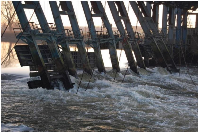
**Figure 104: Damaged weir at Grave and emptying of the section upstream (“Bestand: Stuw Grave”, 2020)**
