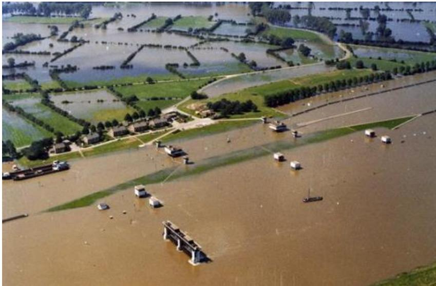
Figure 18: Zero gross head Sambeek weir 1980 flood wave ("Hoogwater 1980 sluizen", 2020)
