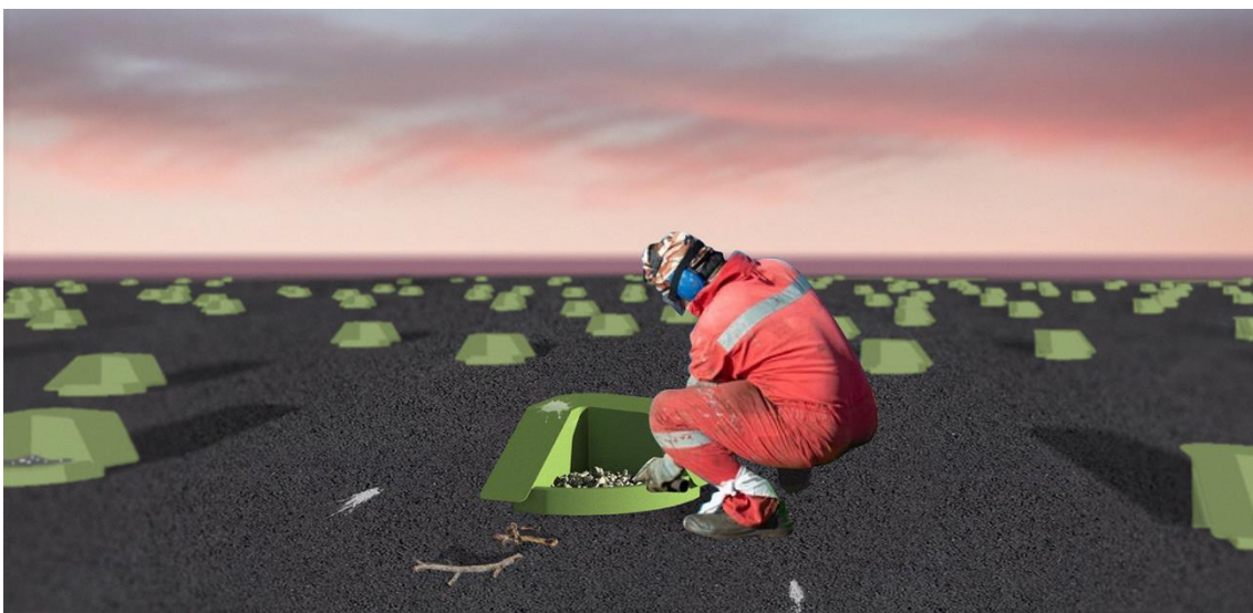
Figure 9 A maintenance worker cleaning an Avian Roof and Nesting Hubs at the end of the breeding season. Source: J. van der Leun.
