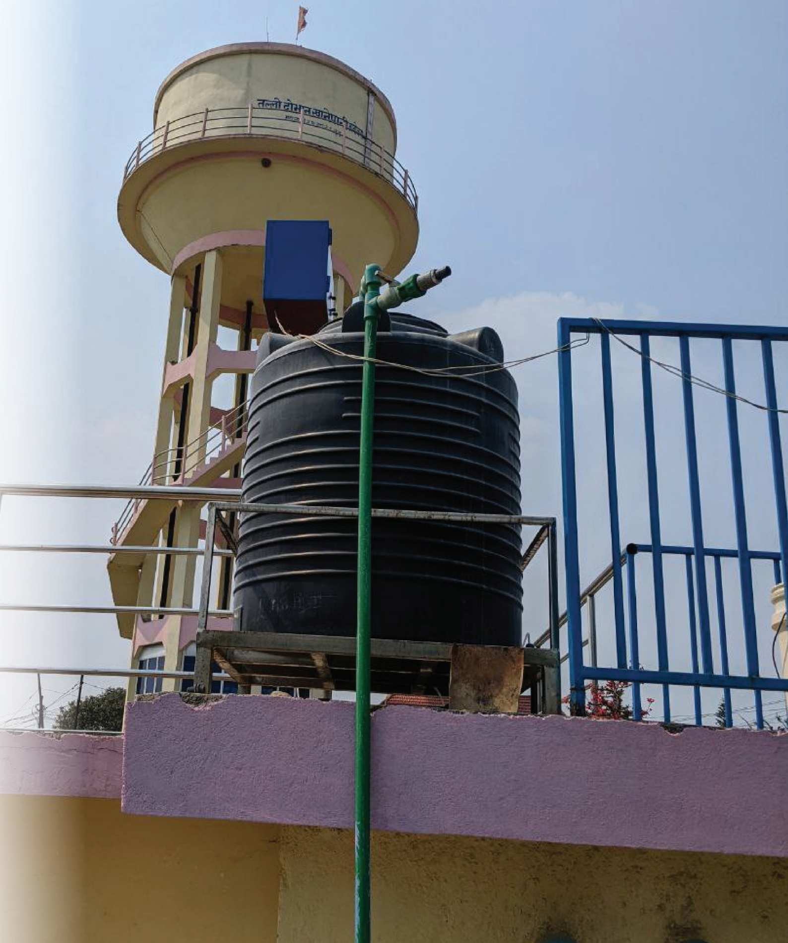
The water tower and chlorine mixing vessel at the Lulu water treatment co-op in Kathmandu, Nepal
