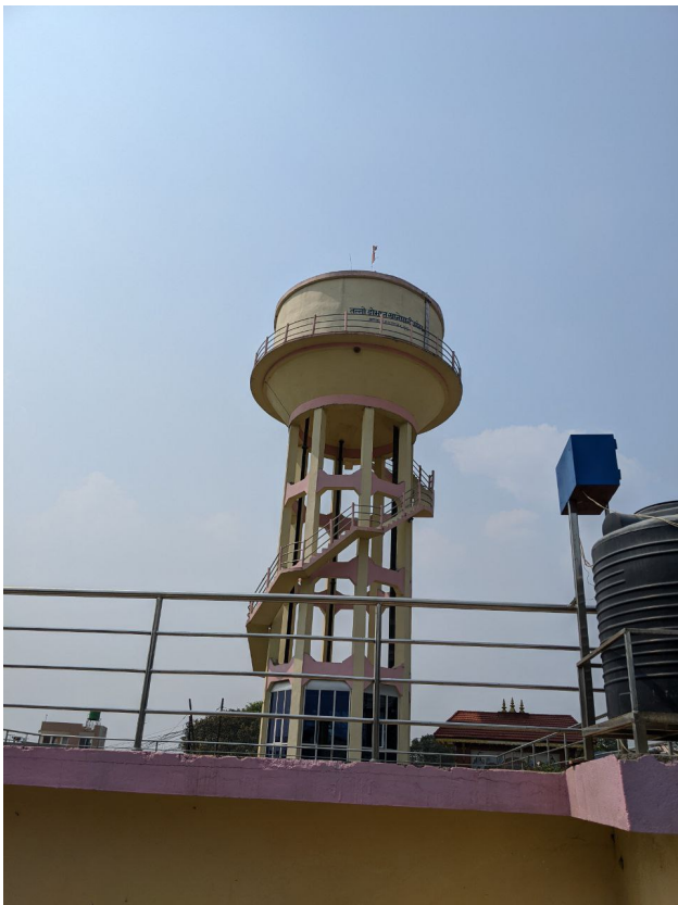
Main water containment tower
