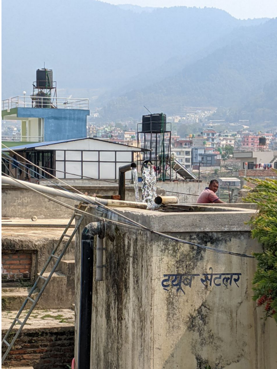
Water flowing into the plant from a collection site
