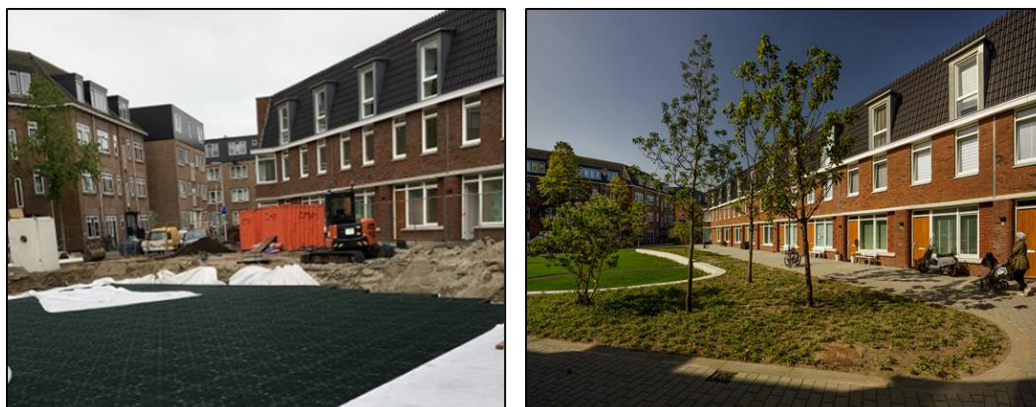
Figure 52 – Staringplein during renovation works (left) and after completion (right).
