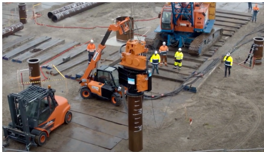
Figure 1: Pile installation at the GDP test site.
