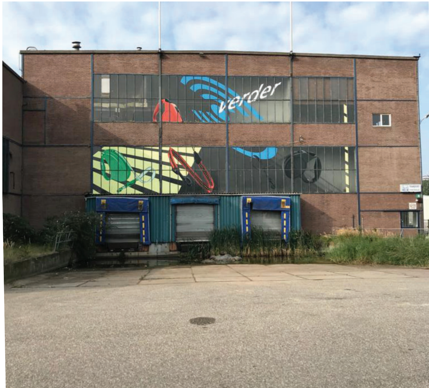
Present front and east facade
