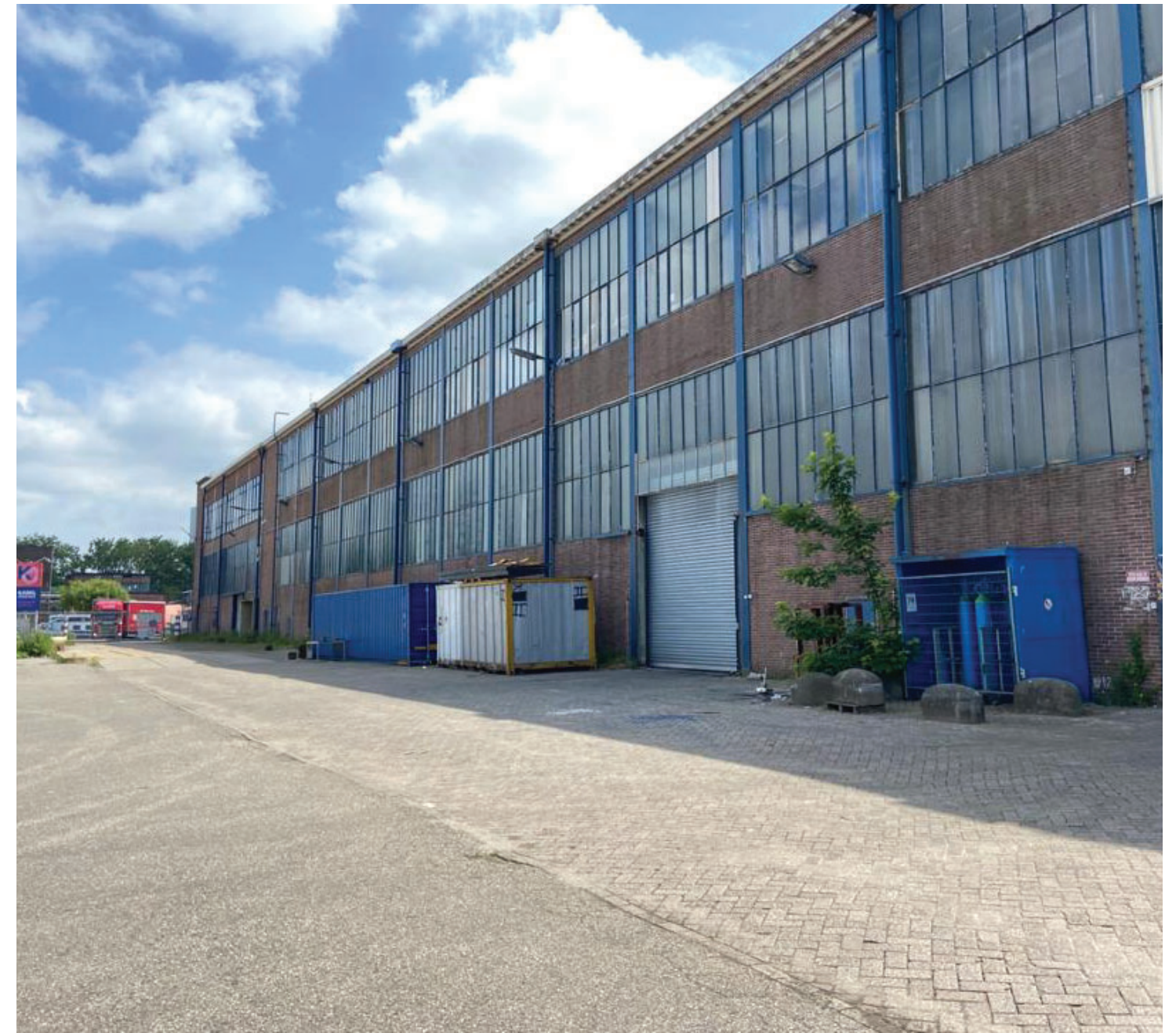
Present, north facade
