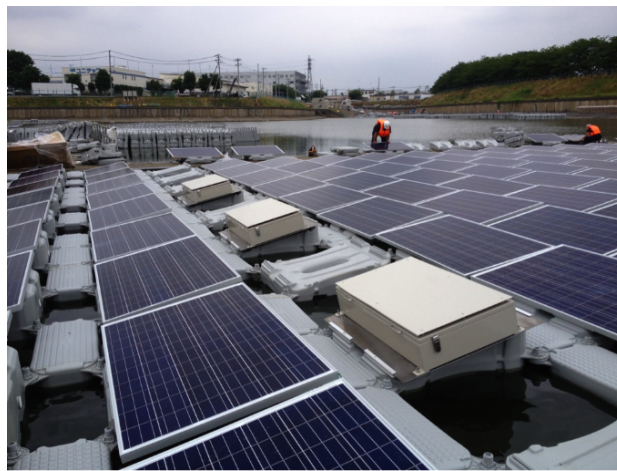
Figure 2.2: Individual raft-based PV at Okegawa via Ciel et Terre [6].
