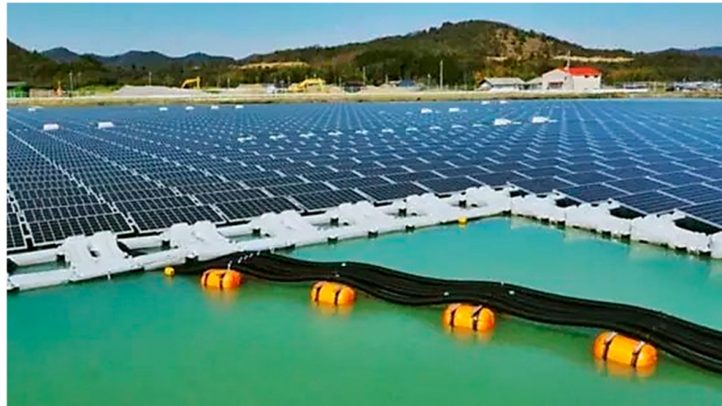
Figure 1.5: Picture of a HDPE pontoon floater design commonly used for large inland FPV systems
