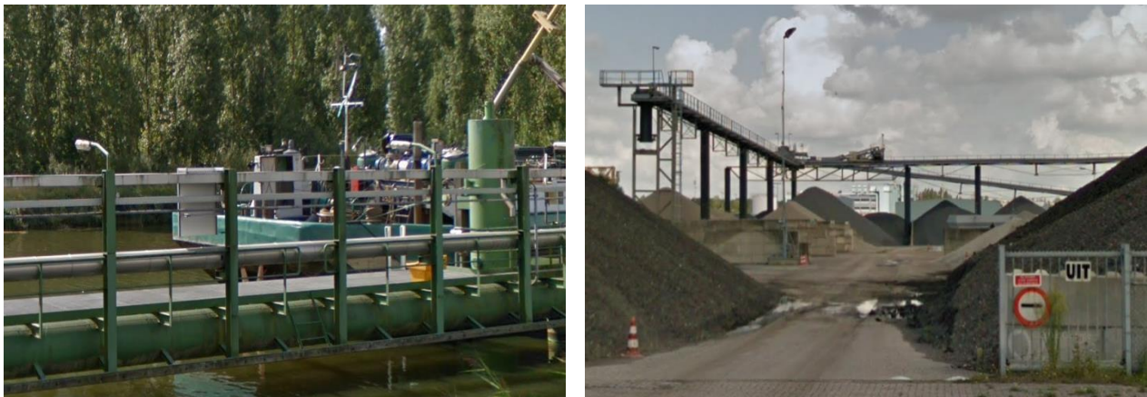
Figure 39: Transport system at the liquid bulk berth (left) and the asphalt plant (right)
