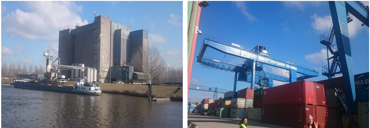
Figure 47: Quay equipment at the agro-bulk terminal (left) and the container terminal (right)
