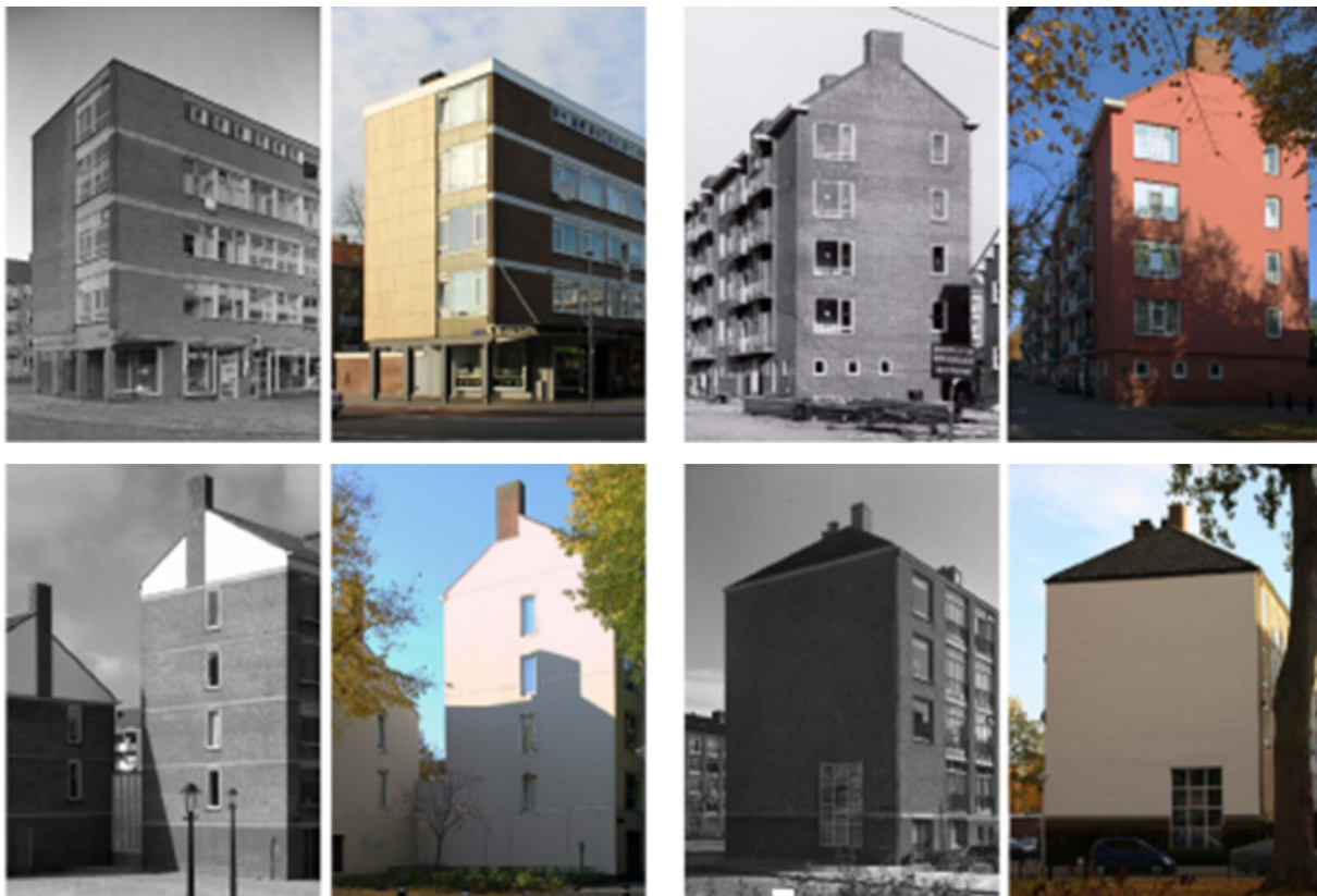
Fig 10. Different buildings where insulation is applied on the outside of the facade, losing the sight of the masonry (Havinga et al., 2020)
