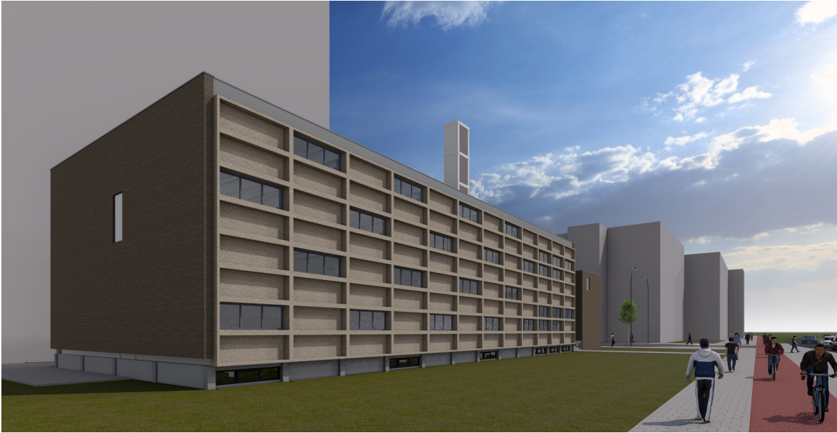
Fig 20. Render of existing facade
