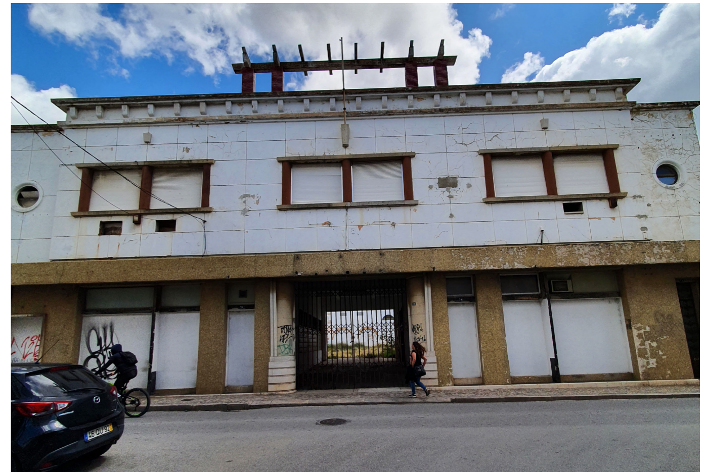
Figure 26: Former EVA building - current state (April 2022).
