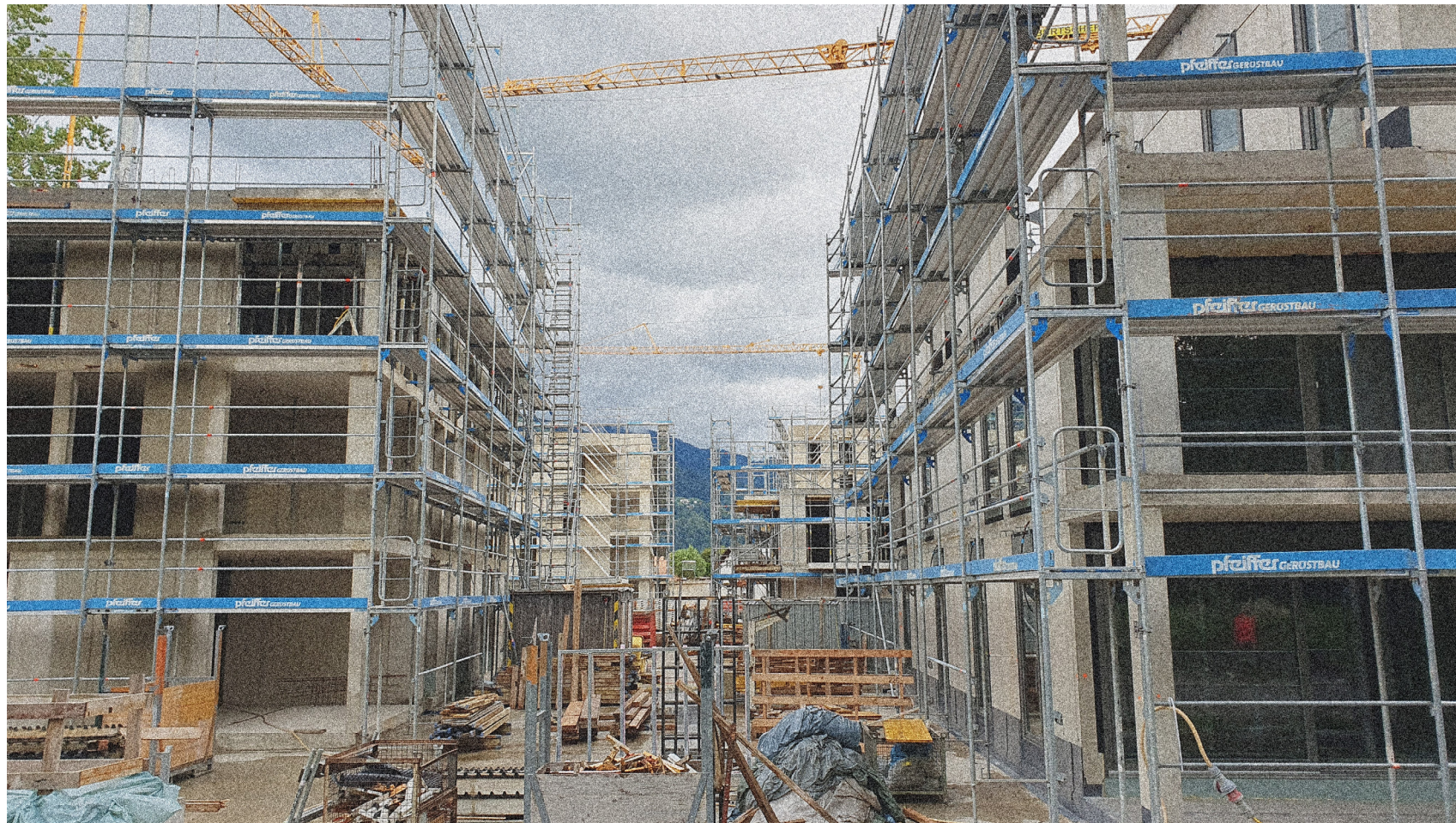
Erection of new residential building blocks in Dornbirn, Austria in 2023.
