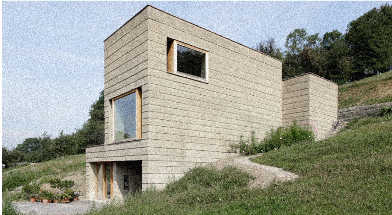
Haus Rauch in Schlins, Austria, made from 100% local soil excavation in 2008.
