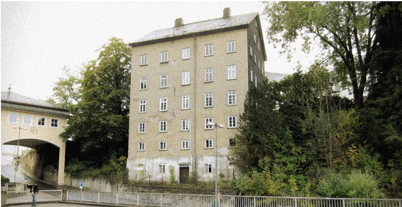
Highest rammed earth building in Germany, built in Weilburg before 1836.
