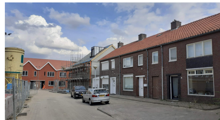
Figure 27 : Picture made during regeneration of Woensel-West. Source: https://www.fotoarchiefwoensel.nl/bouwsloop/oud-woensel/
