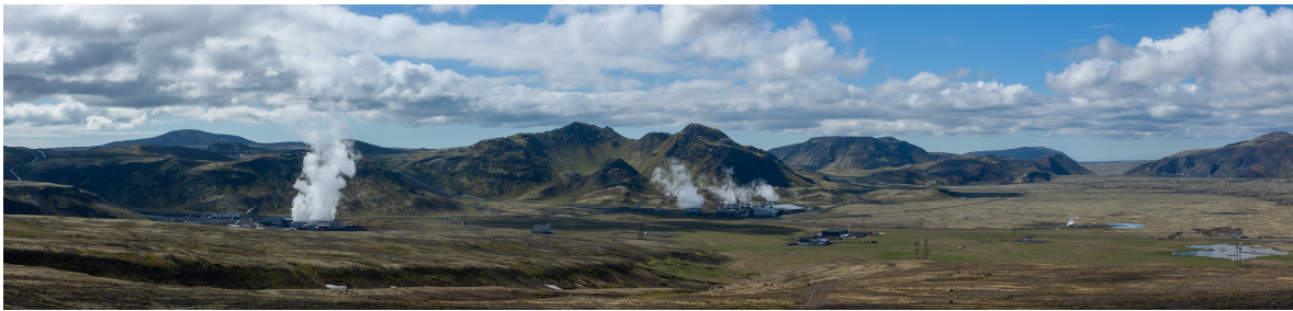
Figure 1: View of the Hellisheiði power plant from the main geophone line.
