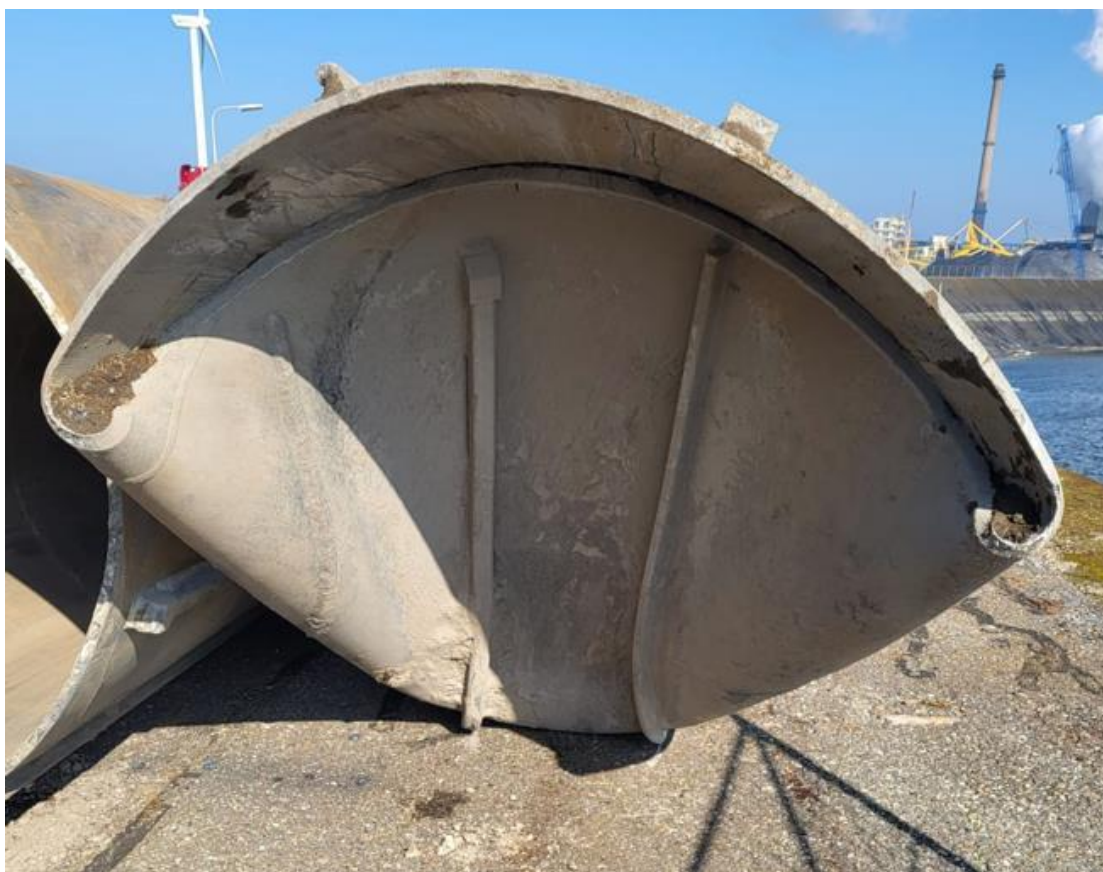
Figure 18 The damaged pile, when pulled out of the soil. Indicating the presence of rock or steel slag significantly larger than the pile thickness (Allnamics Geotechnical & Pile Testing Experts, 2024).
