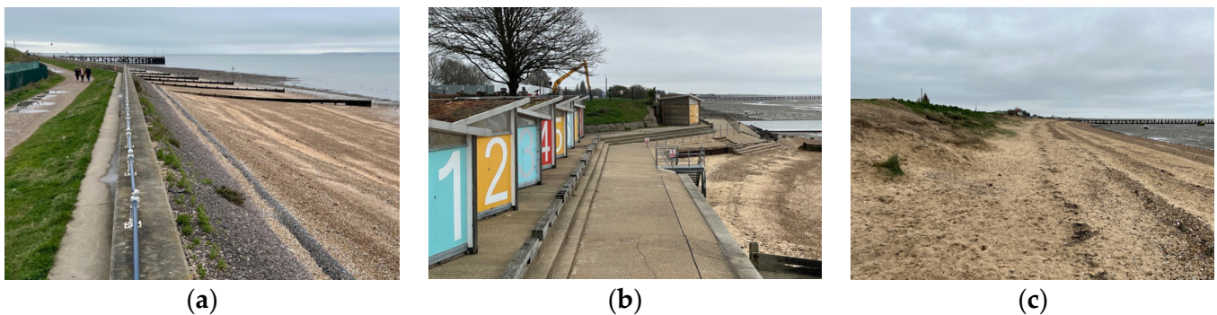
Figure 2. Current coastal defences in Southend-on-Sea (March 2023): (a) vertical seawall in Gunners Park; (b) concrete steps on Rampart Terrace; and (c) sand dunes in East Beach.
