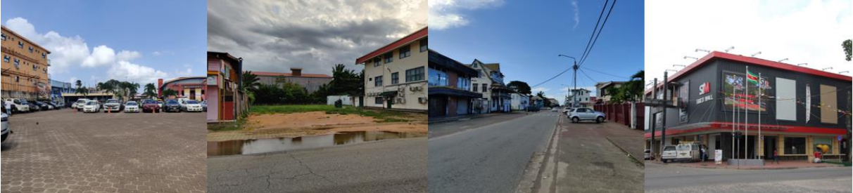
Figure 4-2 Example of parking, vacant lots, wide streets and large roofs in the study area
