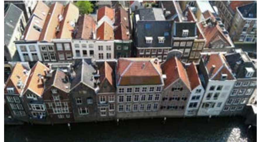
Figure 22. Aerial picture of the dike and main street the Voorstraat.
