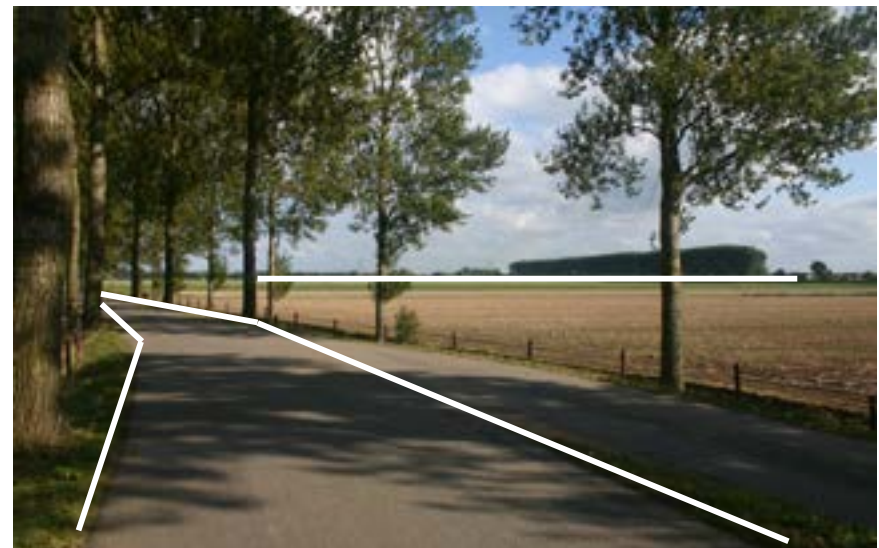
Figure 55. Angles along the dike.
