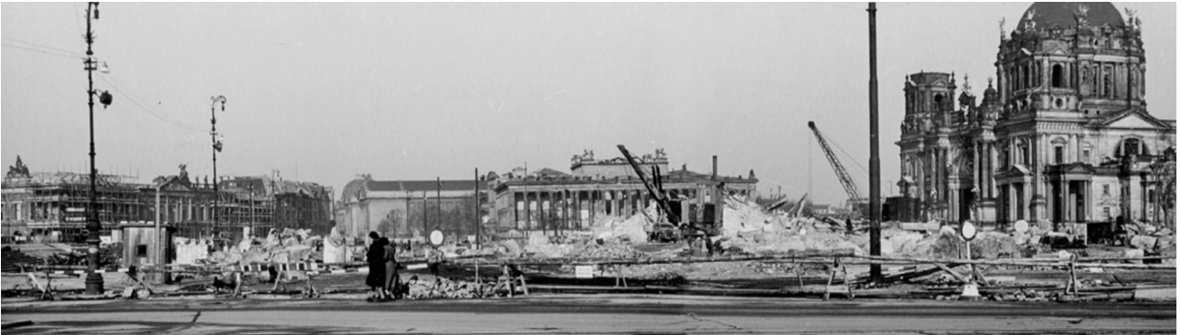
Figure 13: The square after the demolishin of the Berlin City Palace
