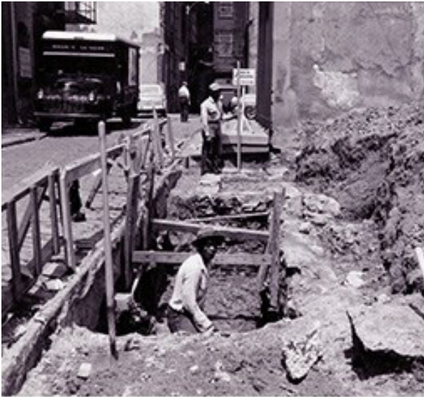
Figure 19: Digging at Franklin Court
