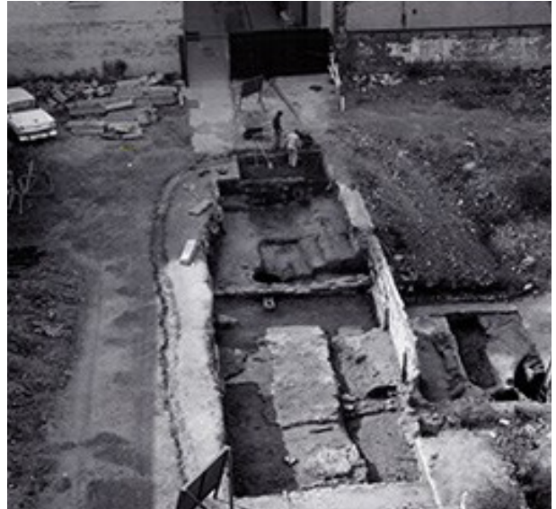
Figure 20: Archeological remains of Franklin Court
