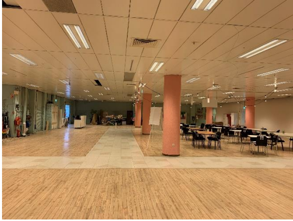
Figure 7 V&D interior, original floors and mushroom columns hidden under lowered ceiling. (Laguna, A., 2023)
