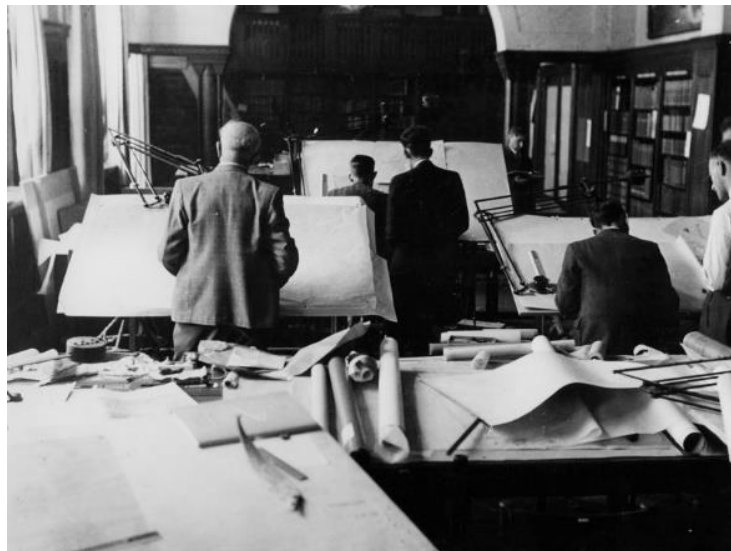
Figure 9. The ASRO and DIWERO working in the municipal library. Stadsarchief Rotterdam, 1940-1942.
