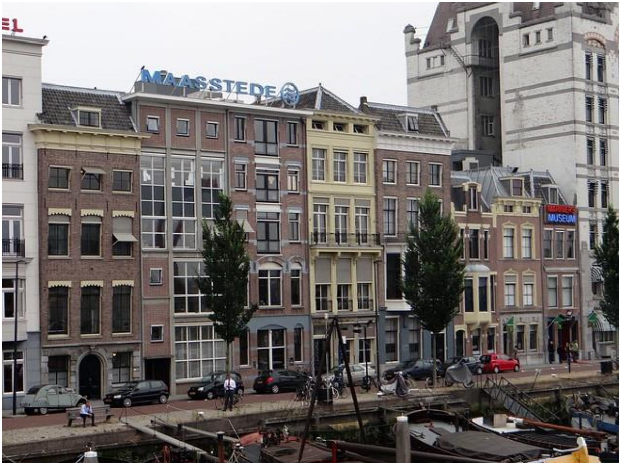
Figure 46. Rebuild merchant houses, Top010.nl, 2013.
