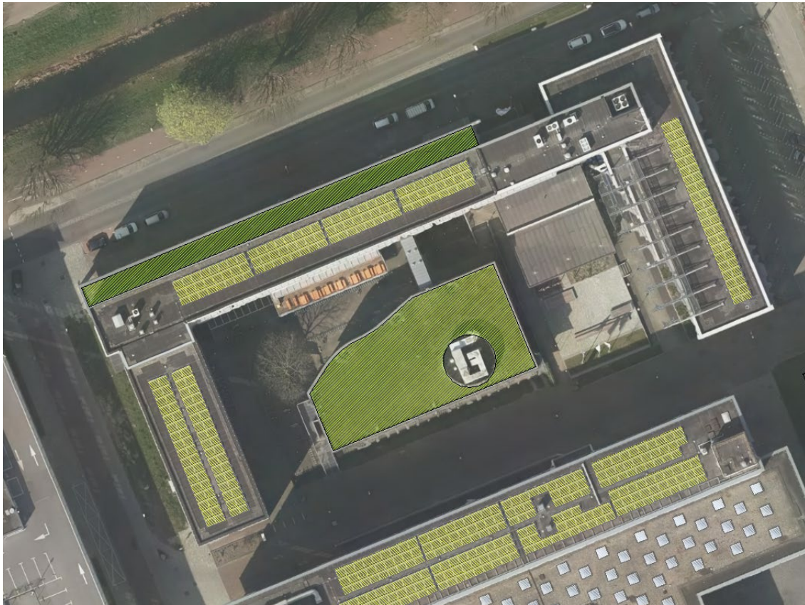
Figure 53: TPM building (31), existing PV and green roofs
