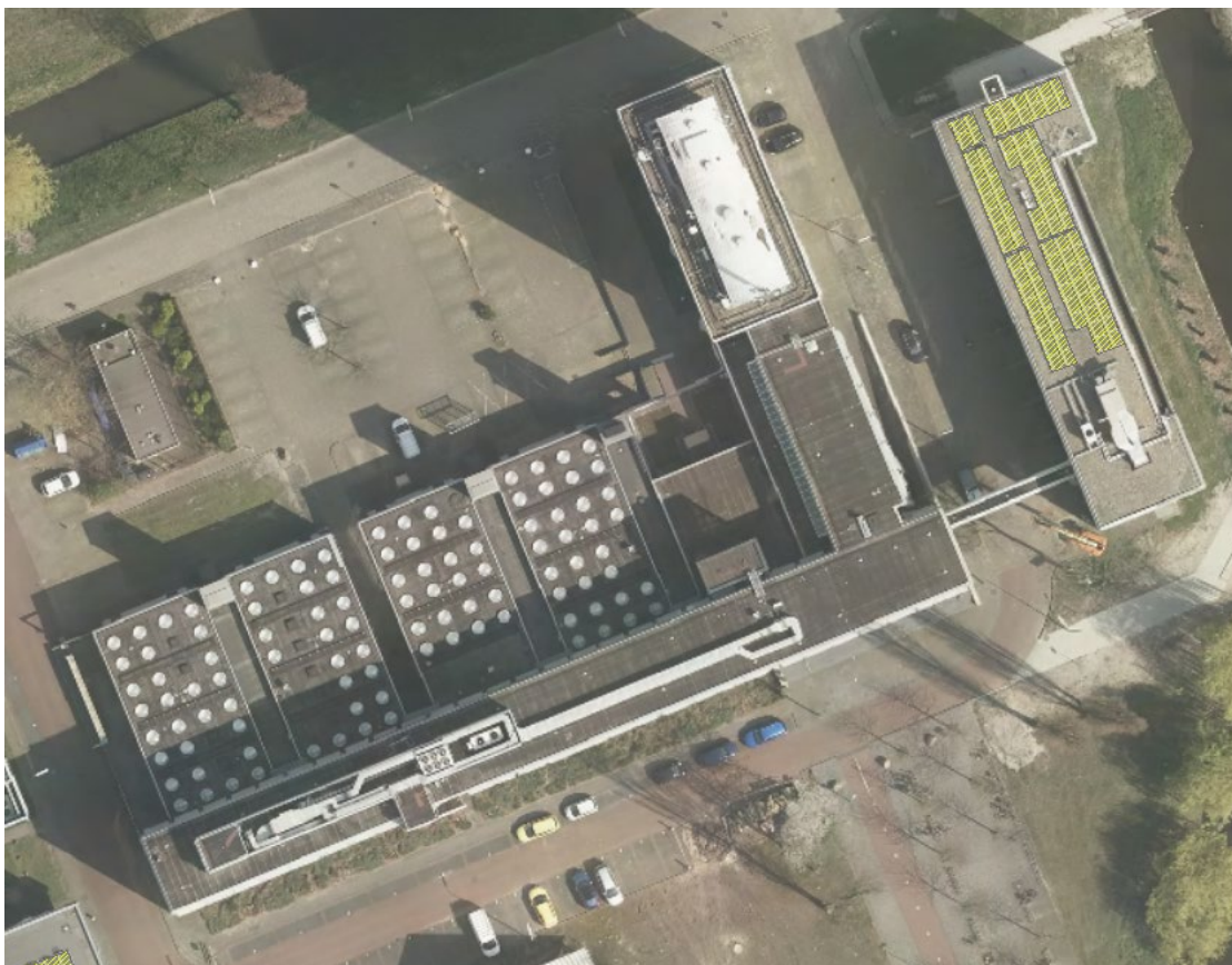
Figure 41: Bouwcampus (26), existing PV and roof lights
