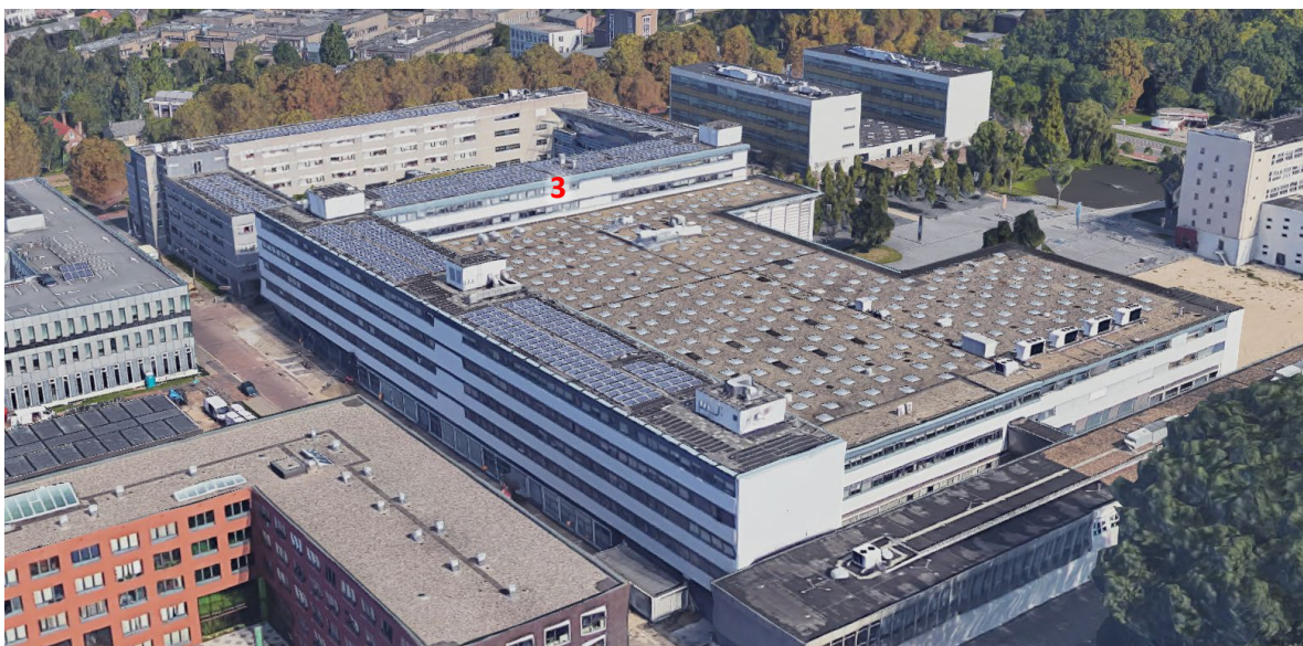
Figure 57: ID building, facade FIDs 3 and 4 highlighted
