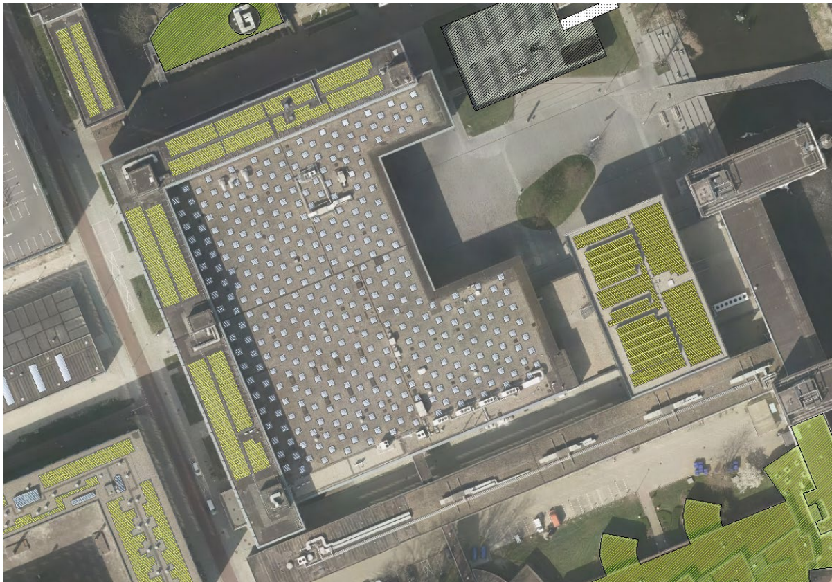
Figure 58: existing PV and roof lights on the ID building (32)
