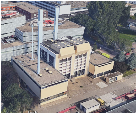
Figure 87 (left): CHP building
