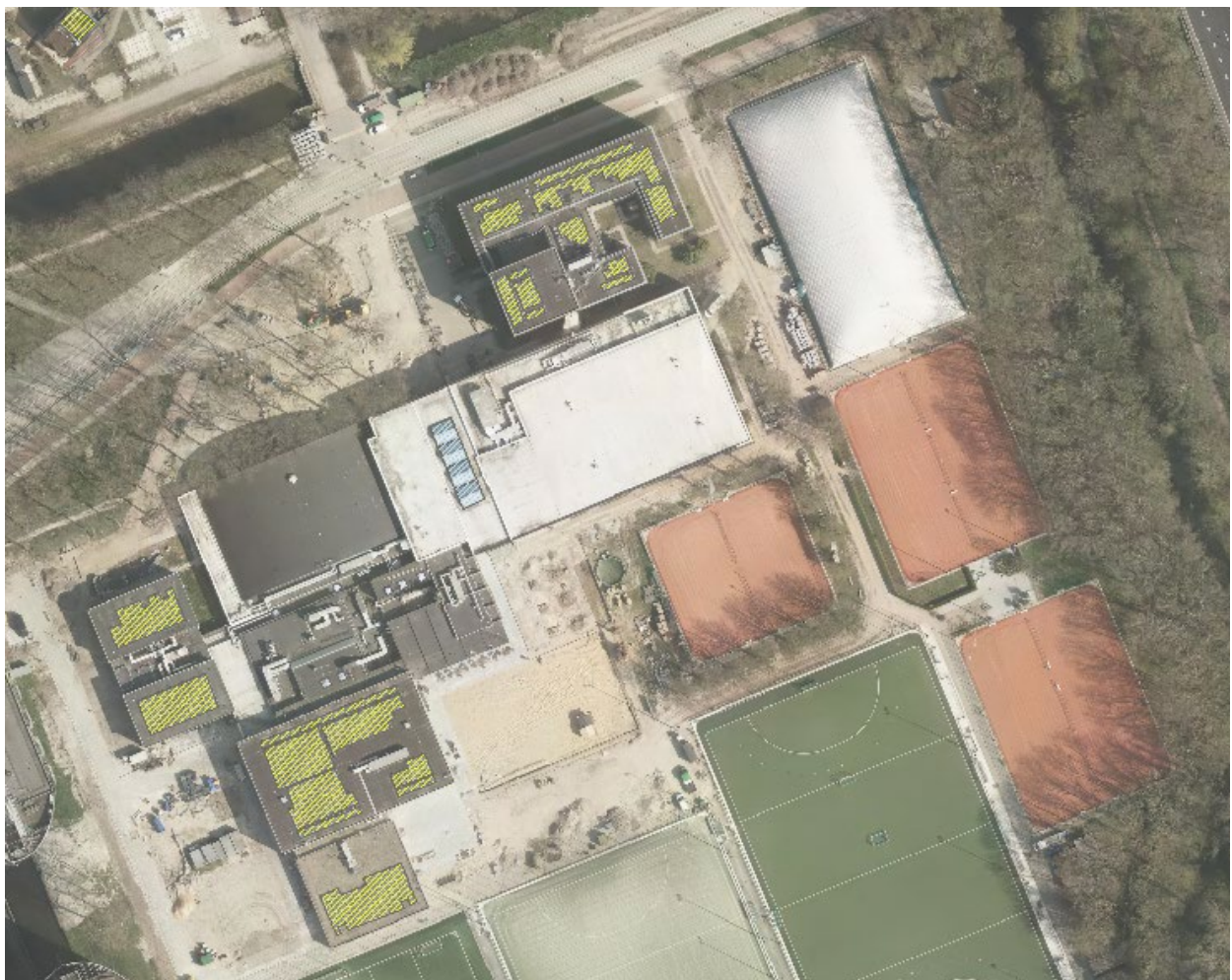
Figure 84: X Delft, existing PV
