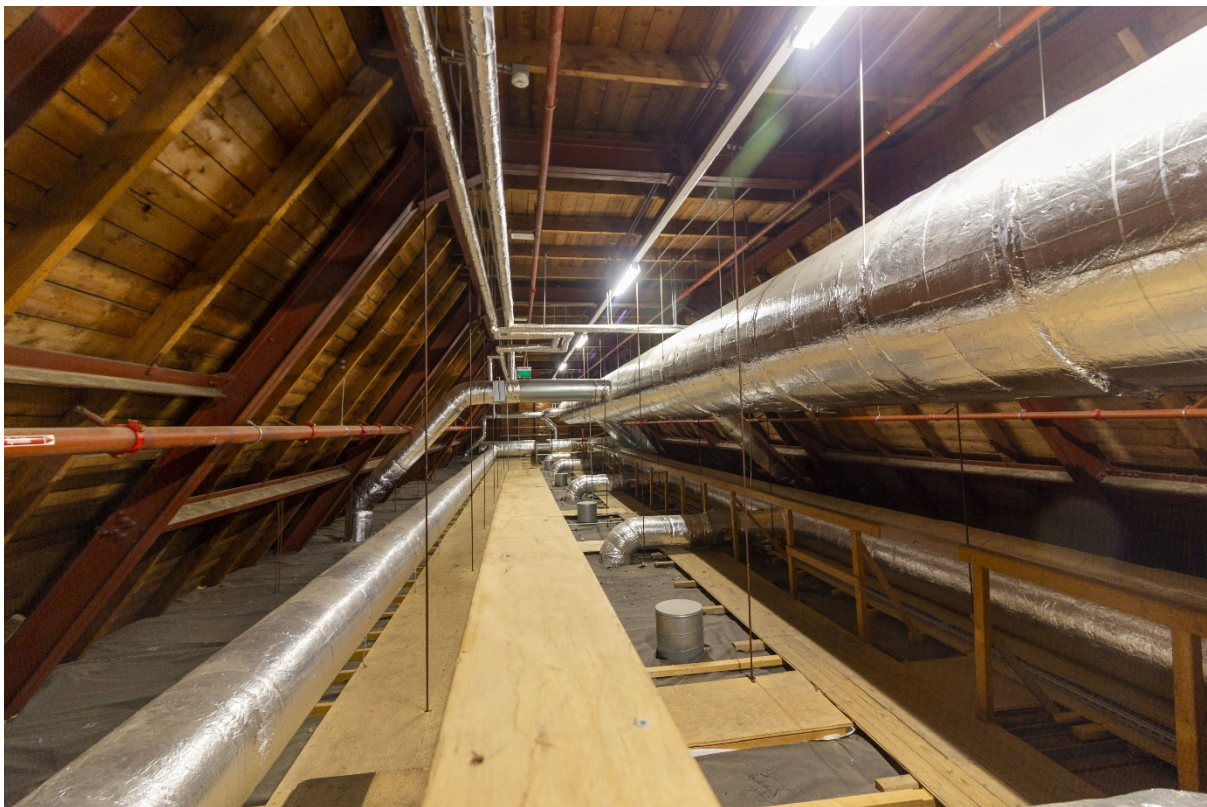
Figure 22: Building 22 roof: steel beams and wood support structure [photo: Michiel Fremouw]
