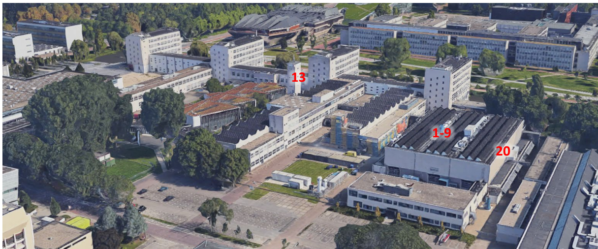
Figure 61: 3mE building (roofs 1-9 and facades 13 and 20 highlighted)
