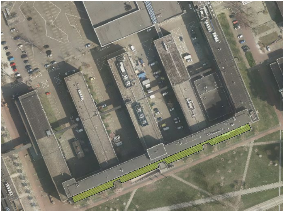
Figure 32: AS building (22), green roof
