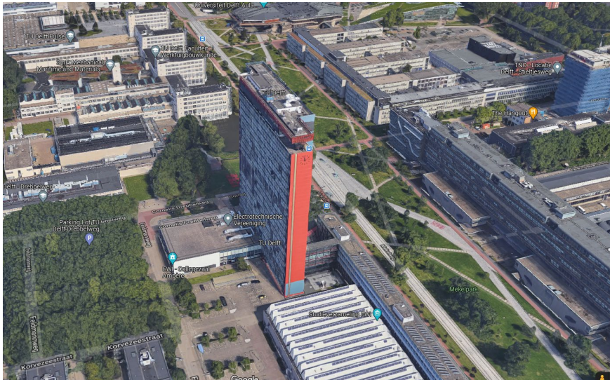
Figure 17: due to the wide spacing between buildings, the EWI highrise only has a limited effect on annual potential.
