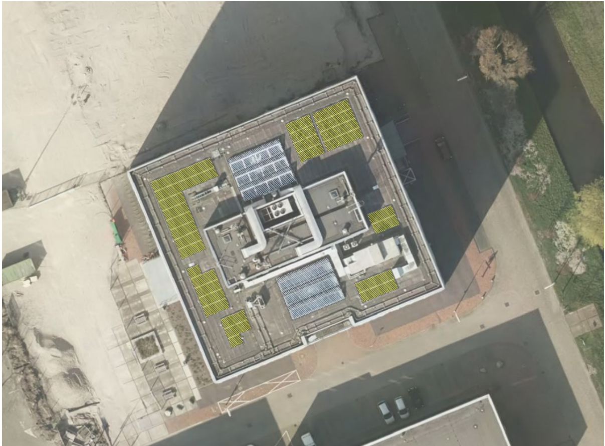
Figure 45: Mathematics building (28), existing PV
