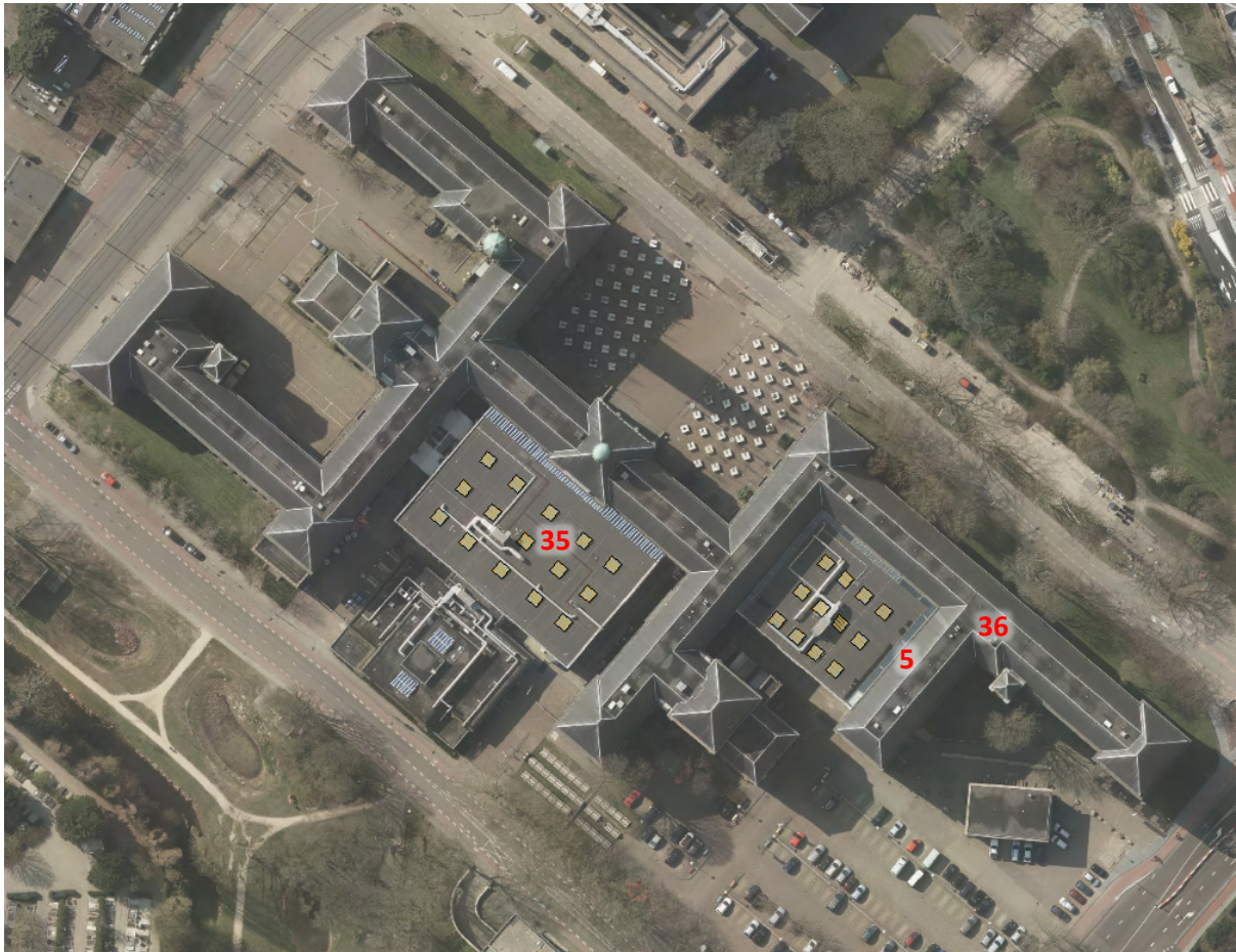
Figure 19: ABE building (8) roof, roof lights and smoke hatches highlighted
