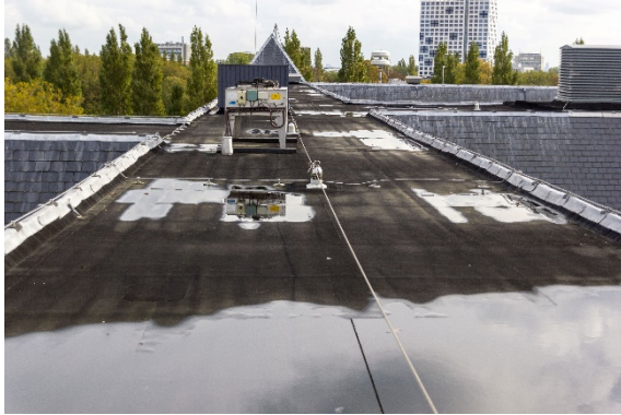
Figure 23 (left): Building 8, flat roof [photo: Michiel Fremouw]
