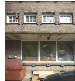
3. Opening provided with new windows
