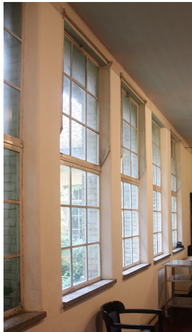
fig. 6.34 Steel windows inside
