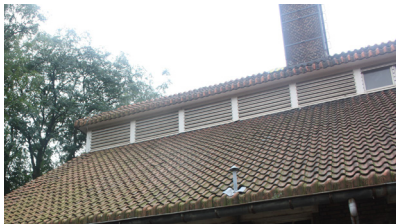
fig. 6.50 Ventilation roof at the disinfection building (12 oct 2016)
