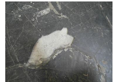
3. Traces of the walls of the changing rooms are still visible on the ground floor. 3. Original floor. Upper layer of the floor with an addition of silicon carbide, resulting in the dark colour of the floor.
