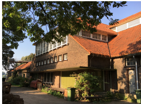
fig. 1.17 West facade disinfection building (T. Sandfort 6 sep 2016)
