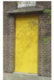
6. New door in existing opening
