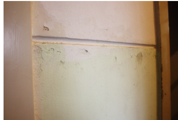
fig. 5.22 Light green plaster below groove (12 oct 2016)
