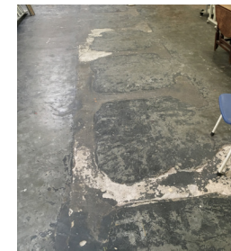
3. Traces of the walls of the changing rooms are still visible on the ground floor. 3. Original floor. Upper layer of the floor with an addition of silicon carbide, resulting in the dark colour of the floor.
