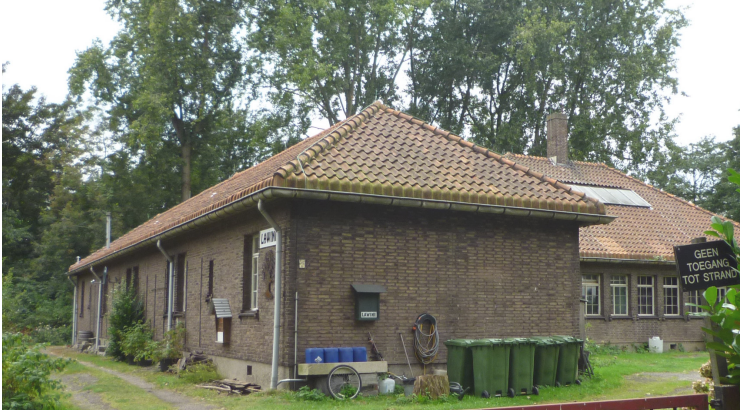
fig. 5.9 General exterior appearance, kitchen building (20 sep 2016)
