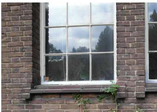
fig. 6.16 Masonry bond around facade openings (sept 2016)
