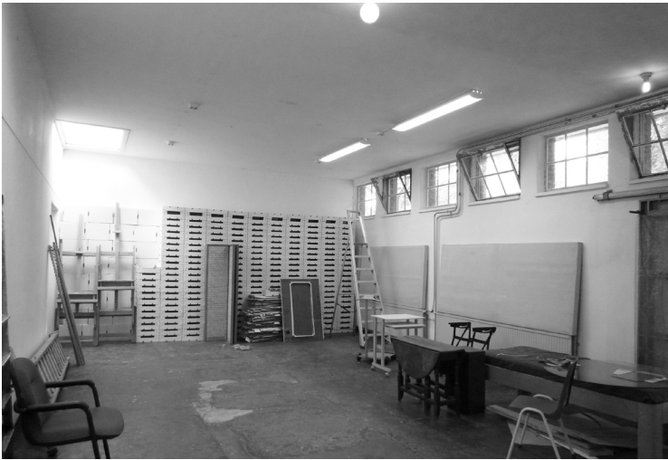
fig. 5.16 Interior space (disinfection building) with high positioned small windows has little relationship with the outdoor space. (20 sept 2016)
