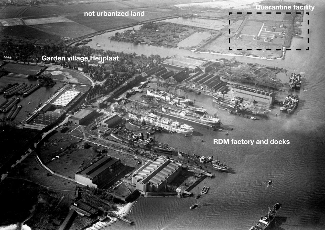
fig. 1.3 Quarantine area short after construction (source: http://www.boijmans.nl/nl/7/kalender/calendaritem/1283/onderzeebootloods/ )
