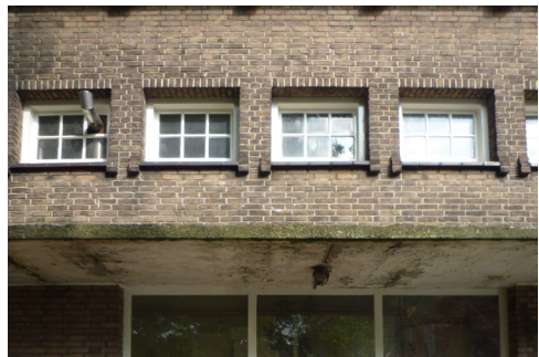
fig. 6.43 Wooden windows in west facade (20 sept 2016)
