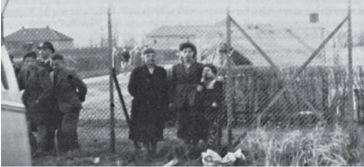
fig. 4.32 Atmosphere of the outdoor space during the accommodation of Jewish refugees, 1938-1939 (source: C.K. Berghuis as quoted in Zwaluw & Hor, 2010)
