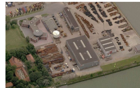
2. Building next to the quarantine area
