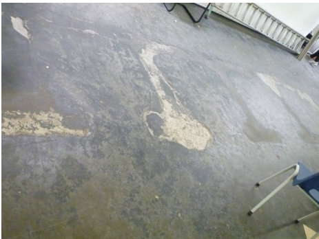
fig. 1.16 Traces left on the floor after the removal of the walls of the changing rooms (20 september 2016)
