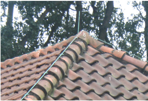
fig. 6.22 Types of roof tiles
