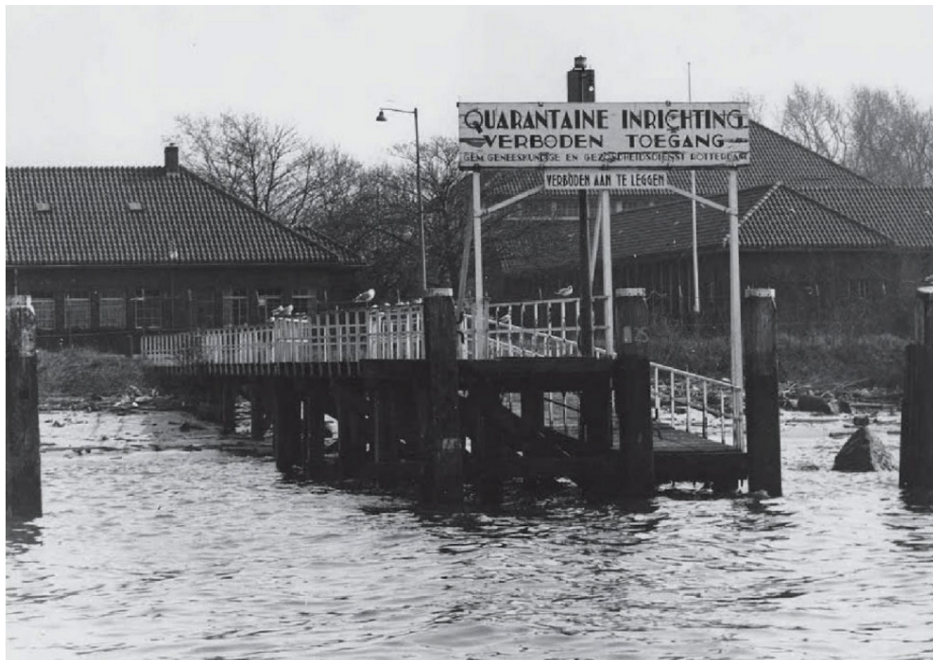
fig. 1.4 The jetty of the quarantine facility (source: Zwaluw & Hor, 2010, p.82)
