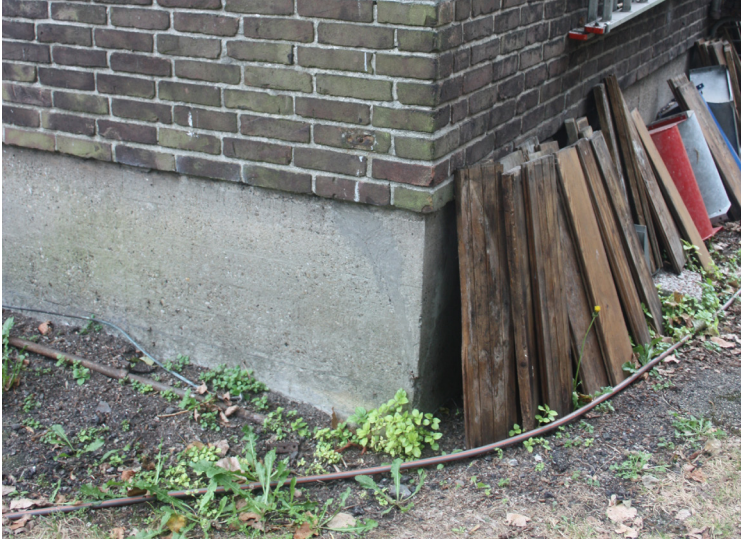
fig. 6.6 Concrete foundation visible above ground level (12 Oct 2016)
