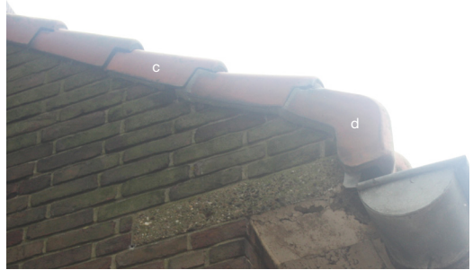
fig. 6.23 Types of roof tiles
