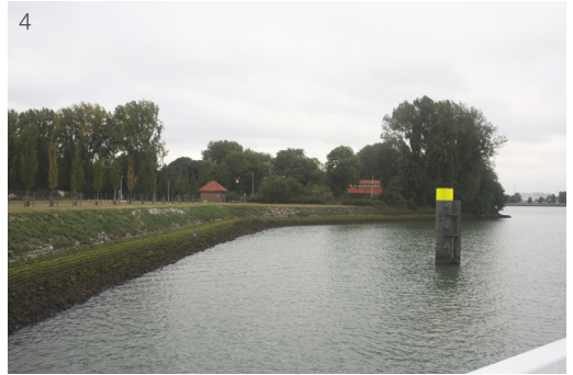
fig. 2.18 Dike along Heysehaven towards quarantine area (12 oct 2016)
