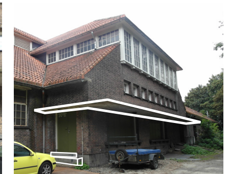
4. Typical accentuating of the entrance with a canopy and stone
