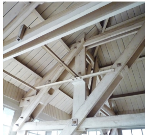
timber roof construction
