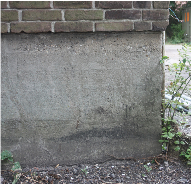
fig. 6.7 Detail of concrete foundation. Lines of wooden formwork still visible (12 Oct 2016)
