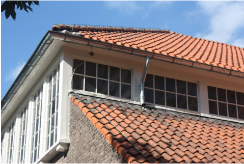
fig. 6.40 Wooden window frames under the roof (9 sep 2016)
