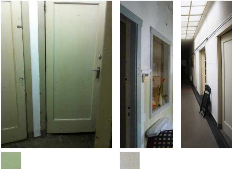
fig. 5.26 Painted timber frames (12 oct 2016)
