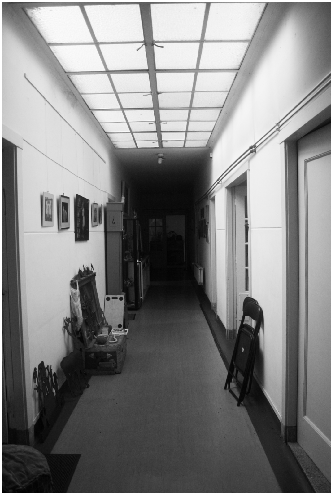
fig. 5.19 Interior view of corridor in nurses home. Natural light is coming from above via windows in the roof an ceiling (12 oct 2016)
