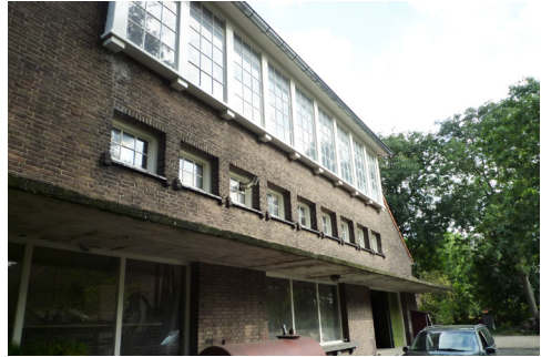
fig. 6.41 Wooden windows in west facade (20 sept 2016)
