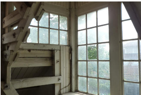
fig. 6.42 Wooden windows inside (20 sept 2016)
