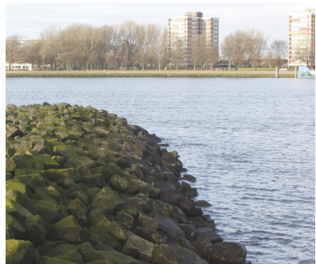
fig. 3.11 Rubble breakwater at the north side of the quarantine area (M. Bijkerk)
