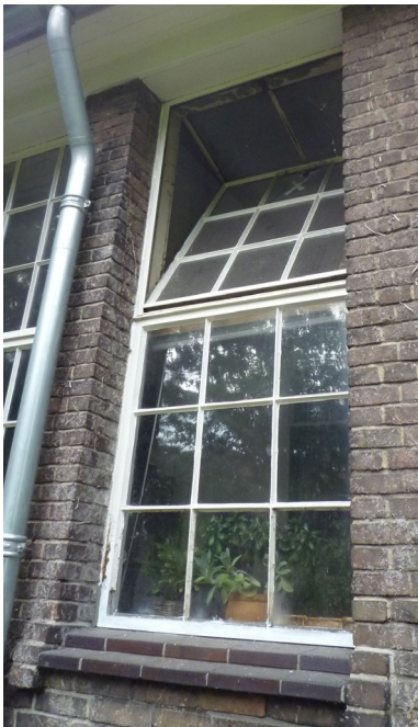
fig. 6.33 Steel windows outside
