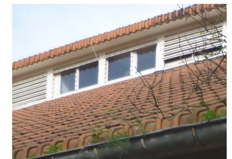
8. Windows made in original segment of ventilation roof
