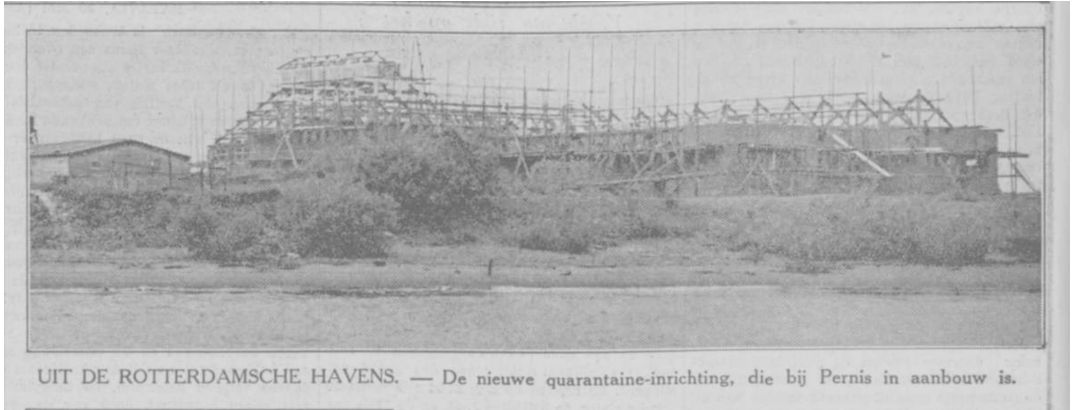
fig. 6.1 Quarantine complex under construction , 1931 (source: De Maasbode, 31 mei 1931, p.4)
