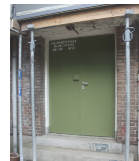
7. Original door: green colour with white lettering (names referring to the function of the buildings).
