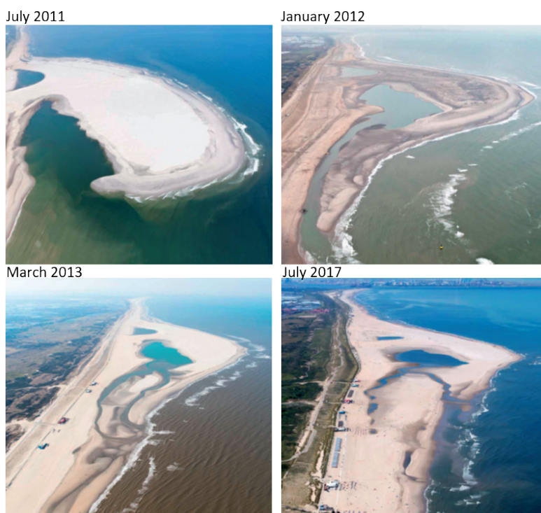
Figure 3. Aerial photographs of the Sand Motor between July 2011 and July 2017.
