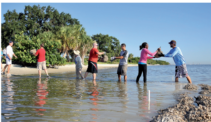
Figure 14. Volunteers place oyster bags at the MacDill Airforce Base project site. Image by Airman st Class Sarah Hall-Kirchner.
