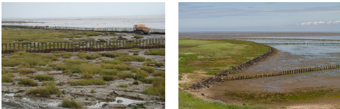
(a) Installation of brushwood fences.
