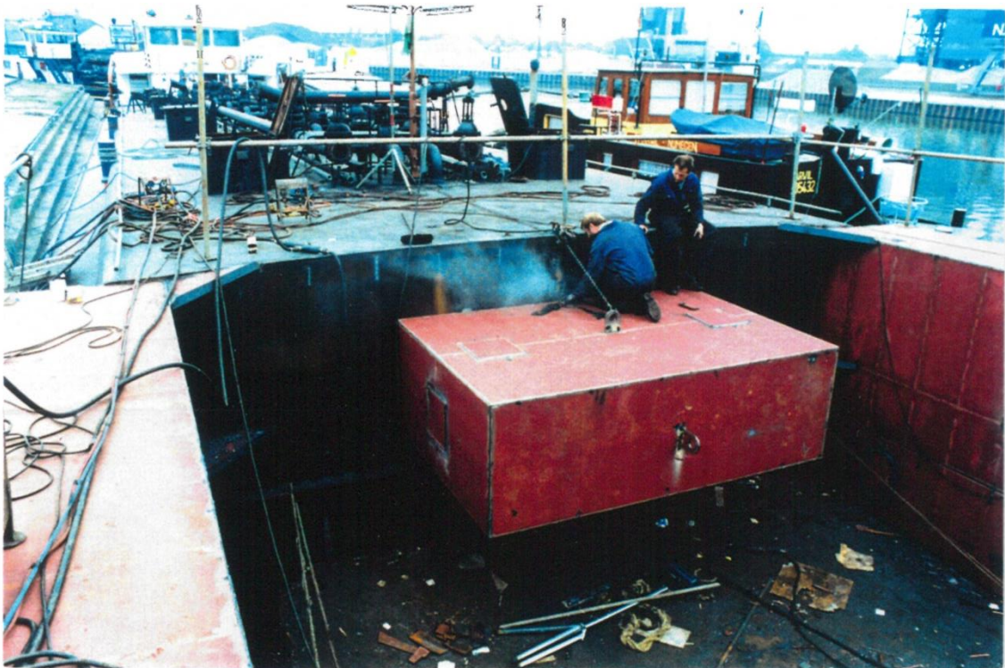
Figure 15 Mounting of the buffer on the Nedlloyd 57. The buffer is added as a precaution; in order to dissipate the ship's kinetic energy that is left after grounding test-section. The buffer is completely filled with foam.
