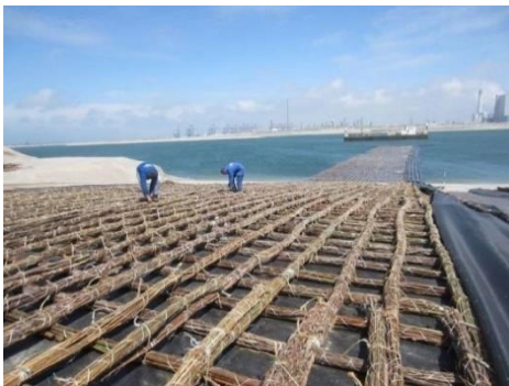
Figure D1: Fascine mattress for use in port (Van Aalsburg, 2022)
